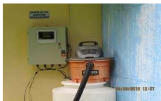
Control Panel and Neutralizing System
