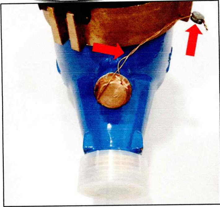
Figure 1. Customized Seal made of copper wire and lead metal
