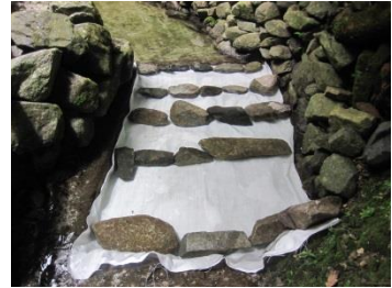
Lapag Mini-Dam 1 (Existing)
